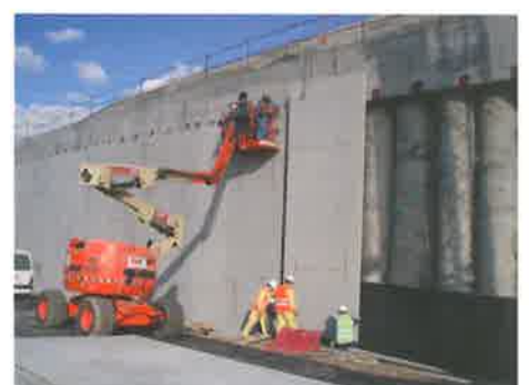
M-50 Highway (Madrid - SPAIN) - Abutment pile coverings
