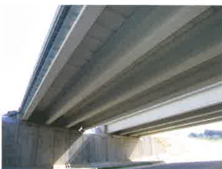
M-501 Road duplication (Madrid - SPAIN) - Buttressed panel abutment
