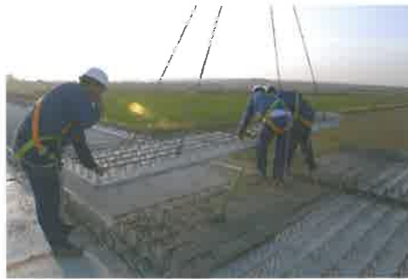
High Speed Train Viaduct - Section Mocejón - Toledo (SPAIN) - Truss slabs
