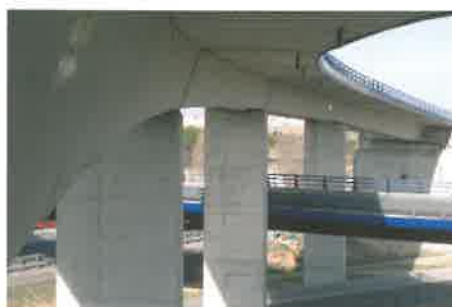
Curved highway connection, from M-45 to A-2 (Madrid - SPAIN), solved with a curved wide 1.50 m high U mono-beam
