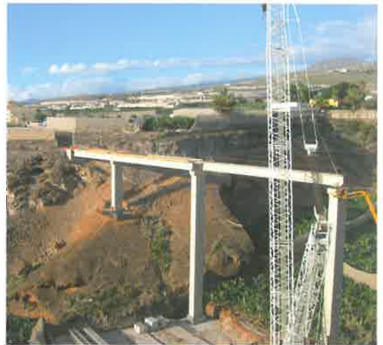
Water and gas pipeline bridge in Adeje (Tenerife, Canary Islands - SPAIN) - Hollow piers; transversal section 1.50x2.20; height 30.0 m
