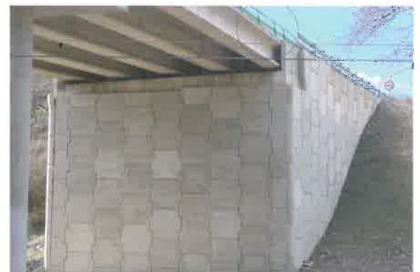
Reinforced earth abutment, supporting I beams
