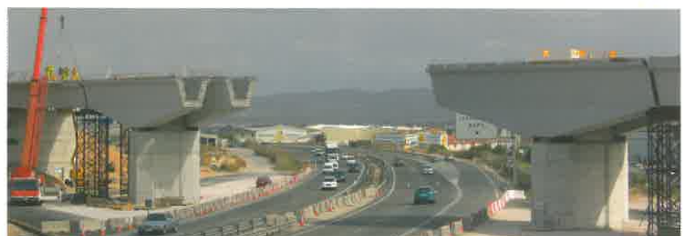
Baladrés Viaduct - Hyperstatic section over A-31 Highway (Alicante) - Spans length: 40 - 62 - 40 - Beam height: 2.60 m - 4.60 m
