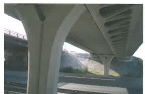
Highway overpass: M-45 over A-4 (Madrid - SPAIN), solved with a wide 1.50 m high U mono-beam Deck width = 15 m - The in situ compression slab is supported at its edges by precast buttresses
