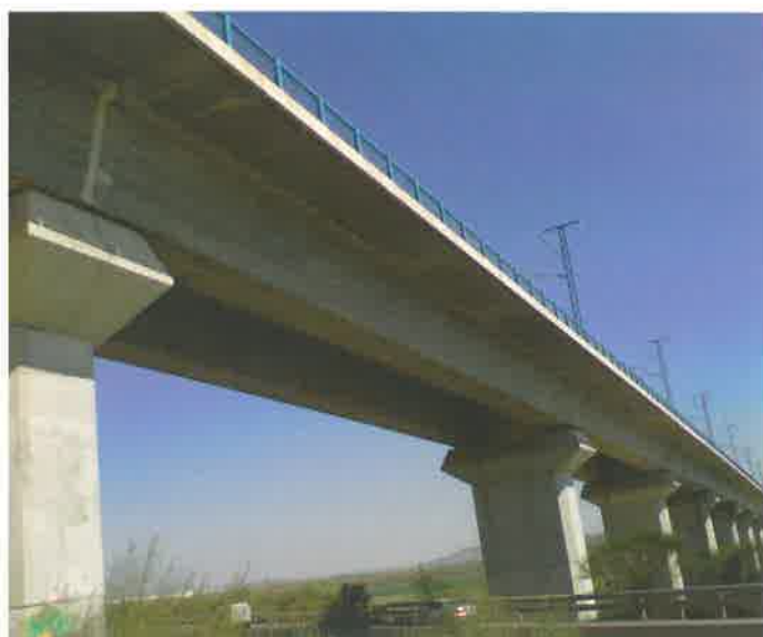
High speed train line Madrid - Barcelona (SPAIN) - Spans length: 30 m - Beam height: 1.90 m - Beam-to-beam joint detail
