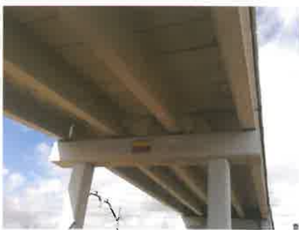
Bridge over Madrid-Guadalajara Railway (SPAIN) 4 IL-110 beams per span
