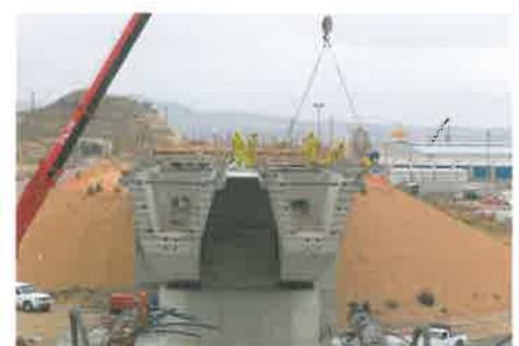
Baladrés Viaduct - Transversal section on top of the piers - Beam height 4.60 m
