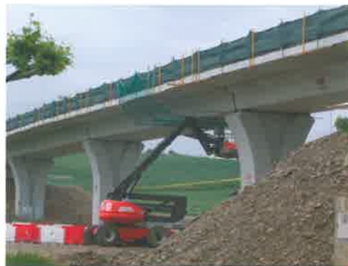
A-12 Highway (Camino de Santiago Highway) - Herviás-Grañón ® section (La Rioja - SPAIN) - Overpass with wide TA-90A mono-beam, supported by palm shaped precast piers
