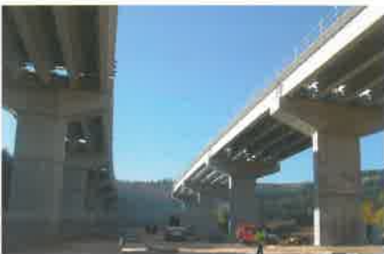
A-67 Highway (Palencia - SPAIN). Section: Alar del Rey – Puebla de San Vicente - Viaduct 2.3 Solution: 5 IP-155 beams per span
