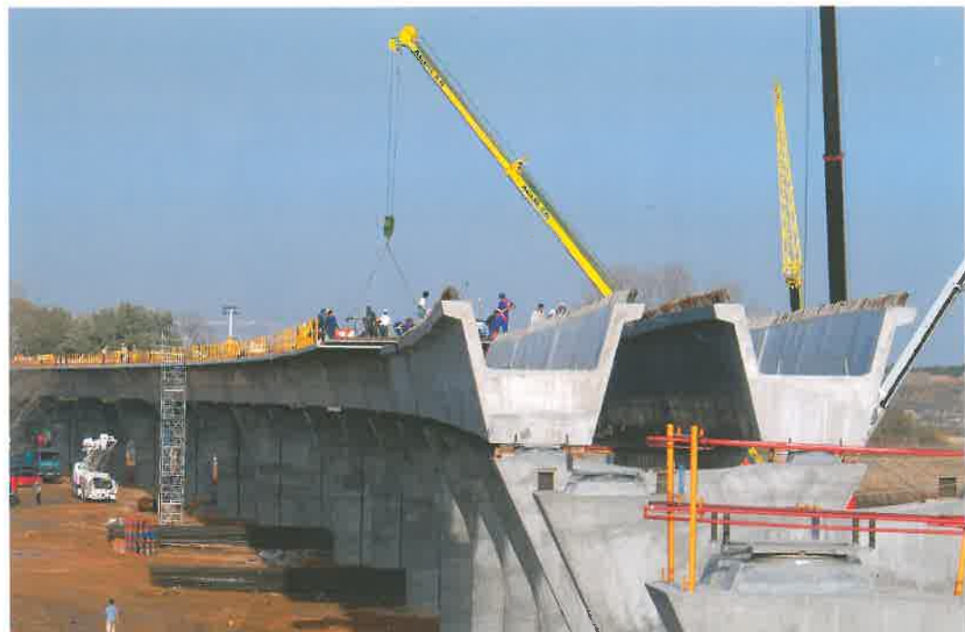
High Speed Train Viaduct - Section Mocejón - Toledo (SPAIN) - Spans length: 36 m - 2 narrow TA-260 beams per span
