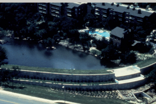
Presa Woodhollow, Texas, EE. UU.
